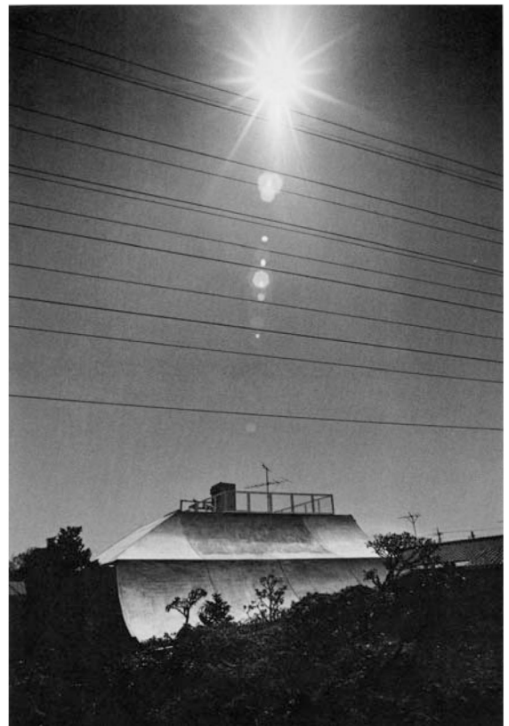
House Under High Voltage Lines (photo by T Oshima)
